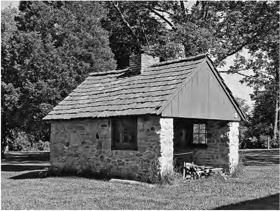
Figure 46. Boone homestead bakehouse, Oley Township, Berks County, Pa., date unknown. Photograph by Philip E. Pendleton. The diagnostic features of a bakehouse are clearly depicted here: solid masonry housing for the oven, chimney, and sheltered work area.
