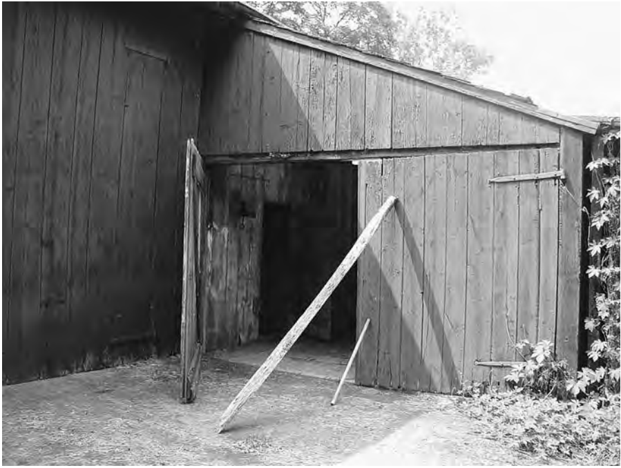
Figure 67. Stoner barn, Lampeter Township, Lancaster County, Pa., c. 1870, east-side horse-power shed. Photograph by Sally McMurry. A “horse power” was a device that allowed horse power to be harnessed to run different types of machines. This horse-power shed was integrated spatially into the Pennsylvania barn, in this instance on the bank side.
