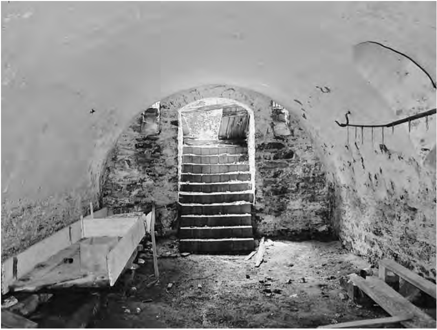
Figure 15. Vaulted cellar, Benedict Eshleman house, Lancaster County, Pa., 1759. Photograph by Sally McMurry. This view depicts the enormous capacity Pennsylvania Germans' root cellars could reach, and the careful workmanship devoted to even utilitarian spaces.
