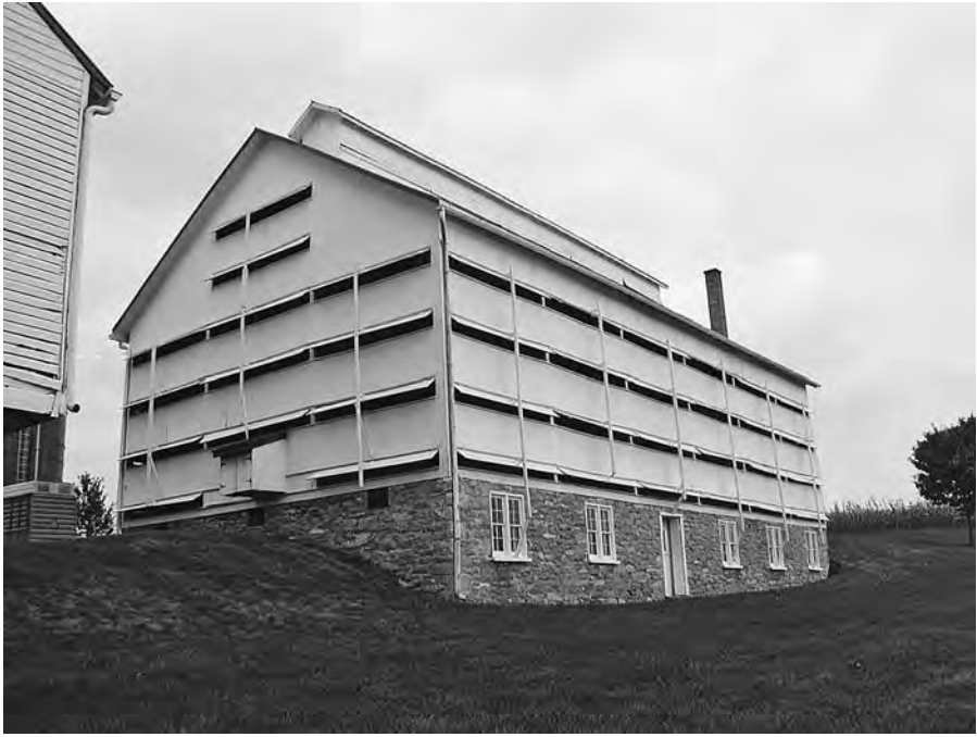
Figure 73. Tobacco barn, Windom Mill farm, Lancaster County, Pa., c. 1875, west and south sides. Photograph by Sally McMurry. A characteristically Pennsylvania German tobacco barn, with banked construction, integral stripping room, and siting within the farmstead complex. The protruding box housed equipment to connect a horse power to the corn barn (just visible at left) via a belt.
