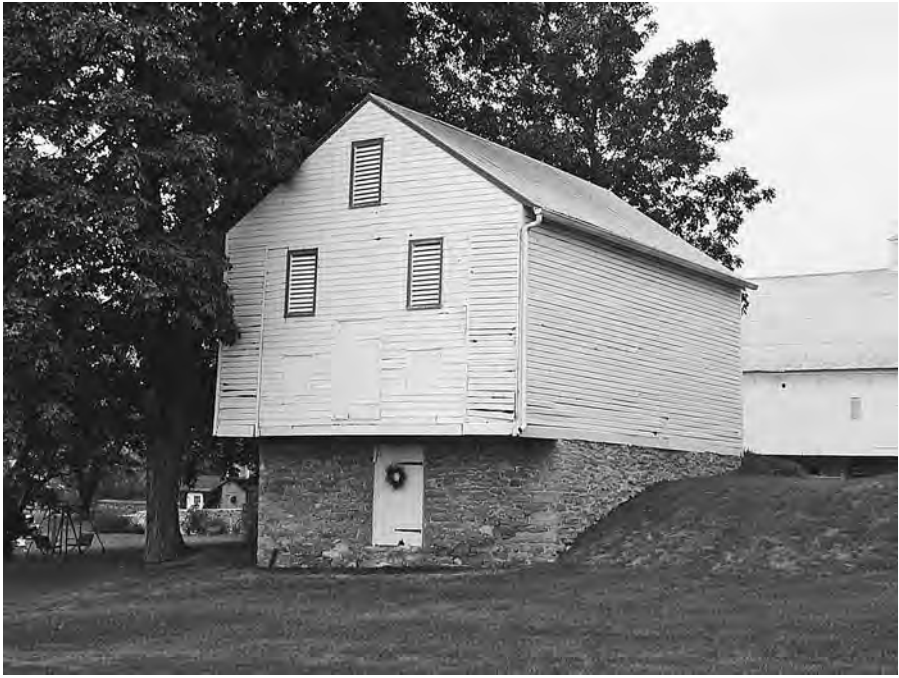
Figure 64. Windom Mill corn barn, Lancaster County, Pa., mid to late nineteenth century, south gable end. Photograph by Sally McMurry. A fine example of a multipurpose building with gable end in the bank. On the upper level, cribs stored corn, and grinding equipment (run from a belt housed in the neighboring building) processed it. The ground level housed machinery. The building nicely illustrates how Pennsylvania German building traditions accommodated mechanization.
