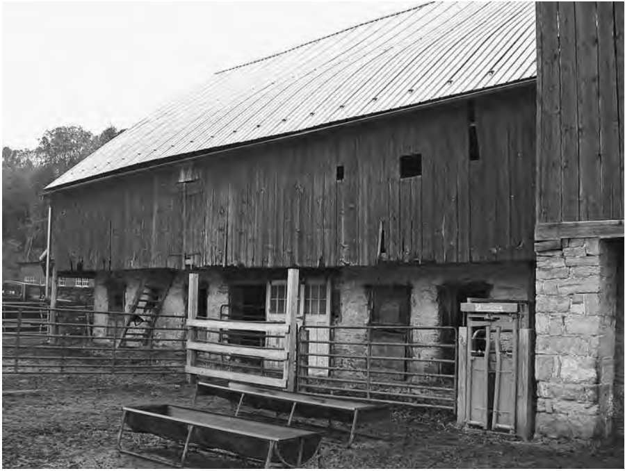
Figure 56. Bertolet barn, Oley Township, Berks County, Pa., 1787, south elevation. Photograph by Sally McMurry. The projecting forebay is clearly shown in this image.
