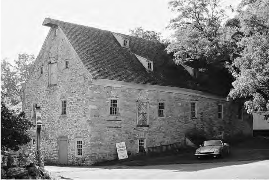
Figure 101. Compass mill, Lititz Run, Lancaster County, Pa., c. 1775, enlarged 1784, north gable and west eaves. Photograph by Diane Wenger. This image shows the banked construction and roadside siting typical for an eighteenth-century mill.
