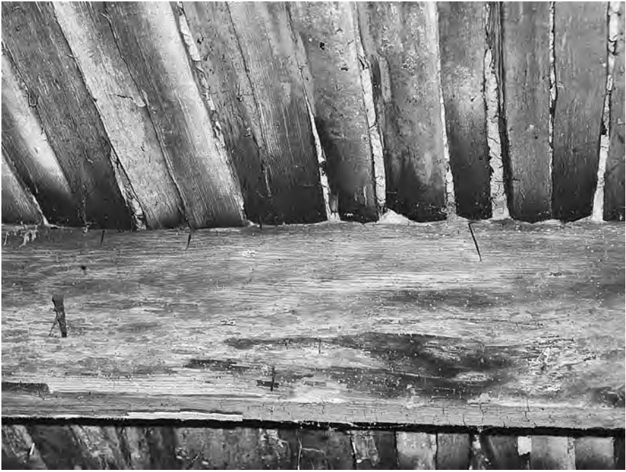
Figure 17. Keim ancillary house cellar, Berks County, Pa., c. 1753. Photograph by Sally McMurry. The gaps in the thin paling resting on the floor joist are filled with insulating materials. This technique was widely used in Pennsylvania German areas.
