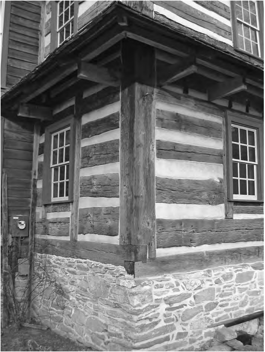
Figure 14. Johannes Hess house, Lititz vicinity, Lancaster County, Pa., mid-eighteenth century. Photograph by Sally McMurry. This corner-post log assembly, sometimes known as Blockstanderbau , shows how the horizontals intersected with a vertical corner post.
