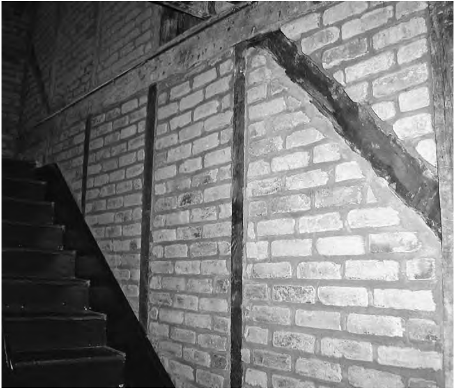
Figure 13. Half-timbering with brick infill, Boalsburg, Pa., c. 1810. Photograph by Sally McMurry. This fachwerk wall reveals a Pennsylvania German aesthetic preference for exposed construction elements.
