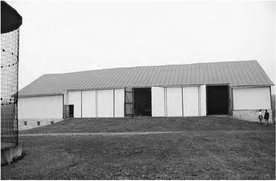
Figure 60. Diller barn, Cumberland County, Pa., nineteenth century, bank side (south). Photograph by Sally McMurry. Each door leads to a separate threshing floor, a visible sign of the complex sharing that often took place on a Pennsylvania German farm.
