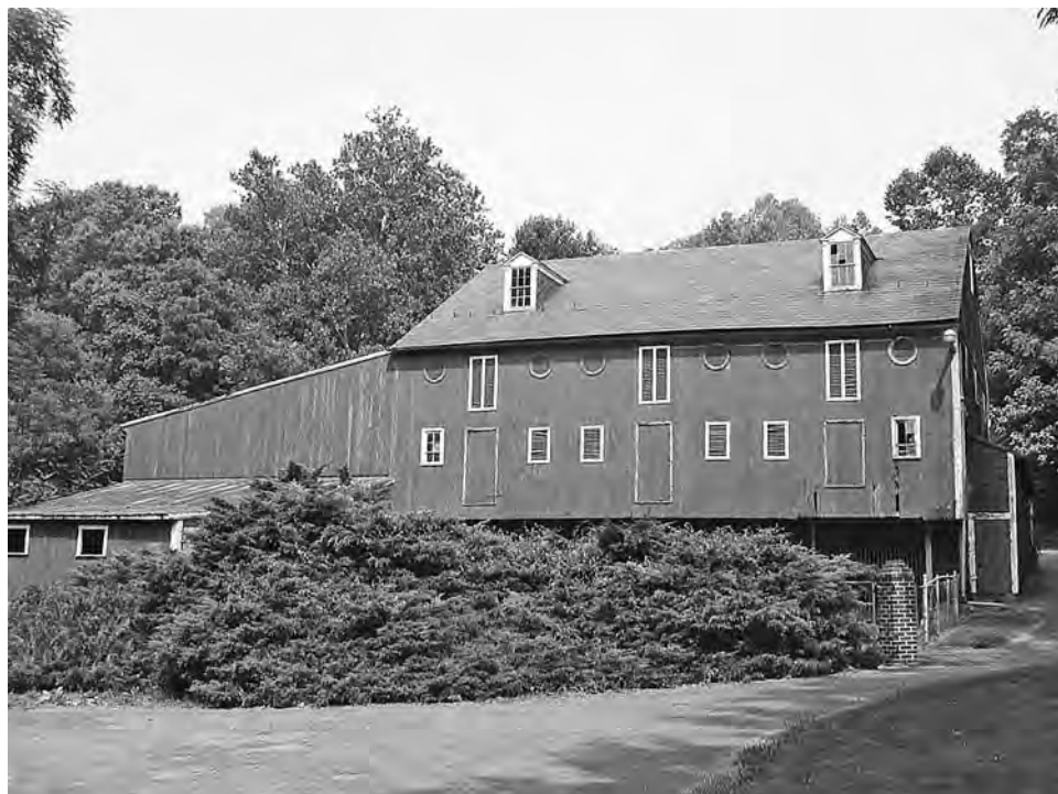
Figure 68. Stoner barn, Lampeter Township, Lancaster County, Pa., c. 1870, west side showing forebay and additions. Photograph by Sally McMurry. This image shows a typical Pennsylvania German barn of the late nineteenth century: made of frame, incorporating ornament, and retaining the diagnostic forebay.
