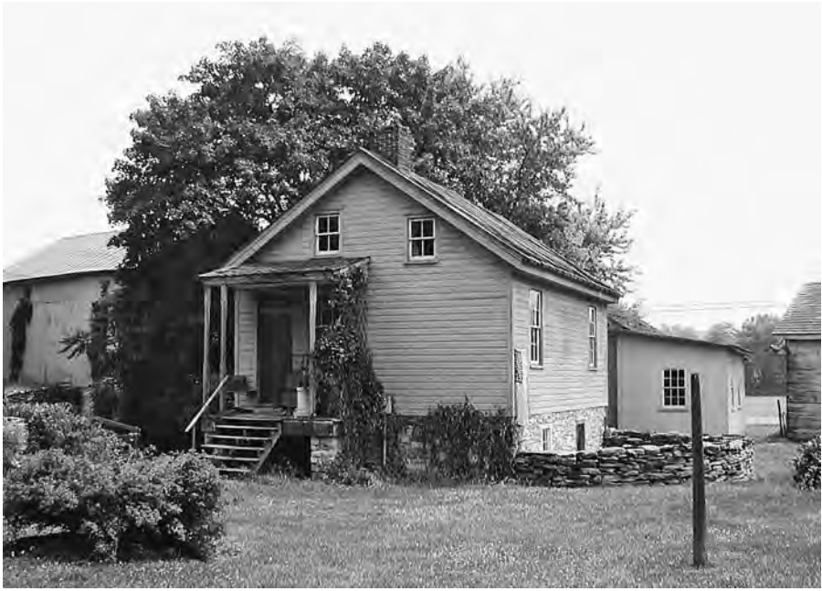
Figure 48. Backenstose summer kitchen and springhouse, Buffalo Springs, Lebanon County, Pa., nineteenth century, north and west sides. Photograph by Sally McMurry. A large spring provides cooling for dairy work on the lower level, while the upper level (accessed from a door in the gable end) housed a summer kitchen.
